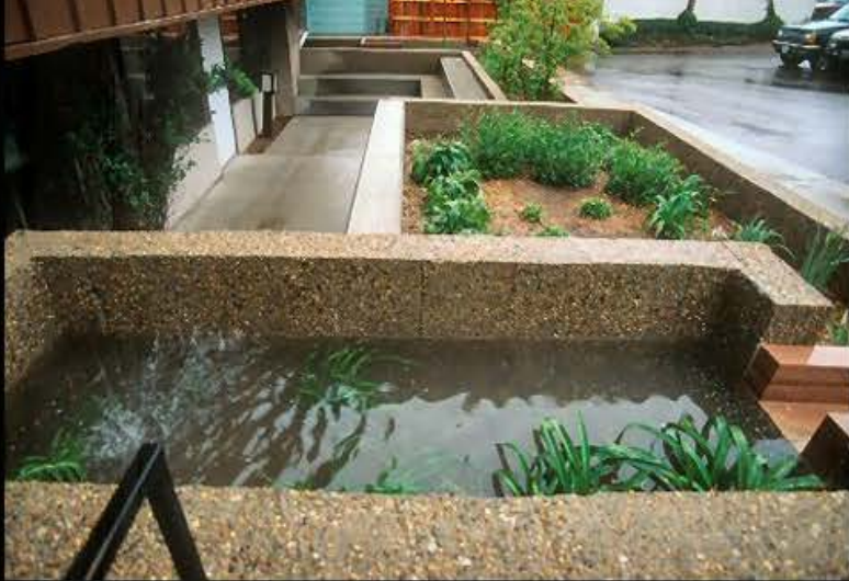
Rainwater collected in planter box then channeled into rain garden Rainwater in painter box then Channeled to rain garden
