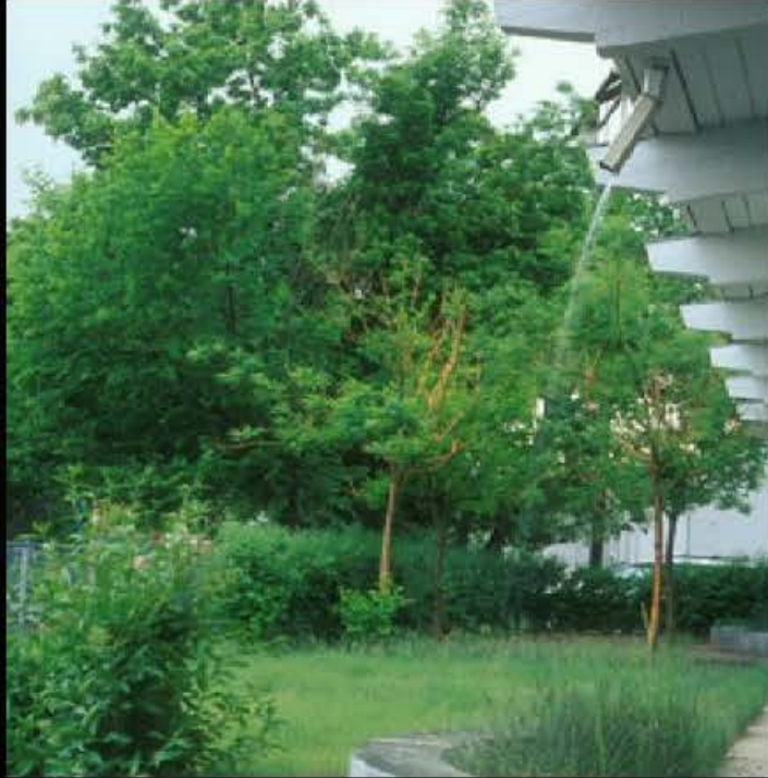
Irrigation by disconnected downspout Denver, CO
